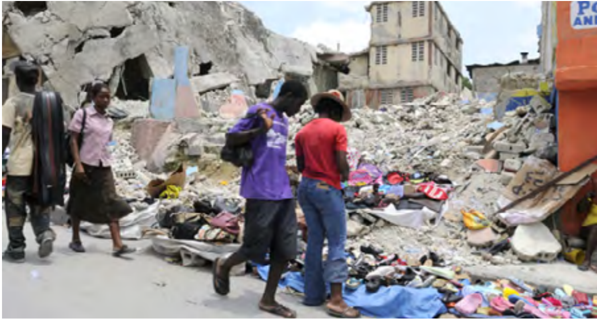
Port-au-Prince, Haiti, August 21: People buying and selling in front of a collapsed building, following the earthquake of January 2010. © arindambanerjee/Shutterstock
